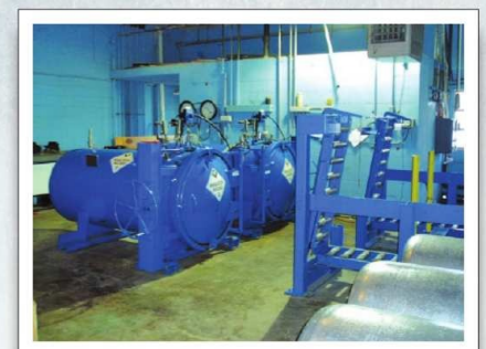
Two one-ton ChlorTainer™ chemical containment vessels were supplied with loaders, scale systems, and instrumentation. Fixed loader system makes for ease of ton container switch out.
