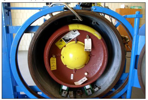
A 1-ton chlorine container is pushed into the secondary containment vessel on rollers. The chlorine transfer hose is attached to the supply valve, pressurized, and tested for any leaks at the hose ends. Then the door is closed, and secured by a clamshell locking mechanism.
