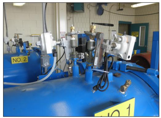
Innovative ChlorTainer $^{\text{IM}}$  cylinder containment vessels are designed for not less than 40 years of service. They enclose chlorine gas cylinders, the chlorine transfer hose, and seismic lock-down brackets. Vacuum breaker regulators are attached for fail-safe shutdown if there is a leak downstream.
