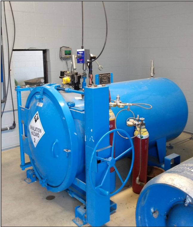
ChlorTainer's failsafe valve is powered open using nitrogen and electricity. If the power is lost, the failsafe valve will cycle closed, and will automatically cycle open when the power is restored.
