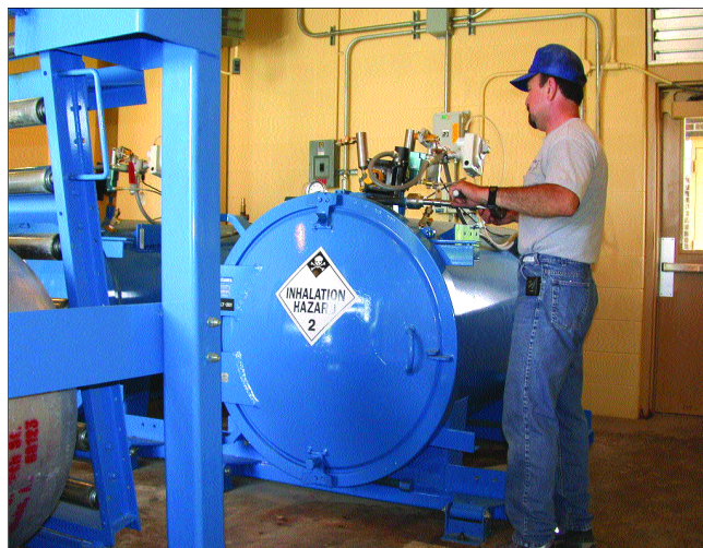
The photo above shows Leavenworth Water Department Operator Mike Domnick tightening bolts on the door of the containment vessel. Mike's comment is that this is the hardest part of the operation, by which he means the entire process is relatively easy.
