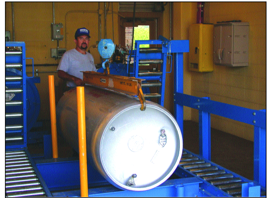
Mike Domnick, Leavenworth Water Department, moves a one-ton chlorine cylinder into place to be loaded into the utility's new ChlorTainer containment systems.
