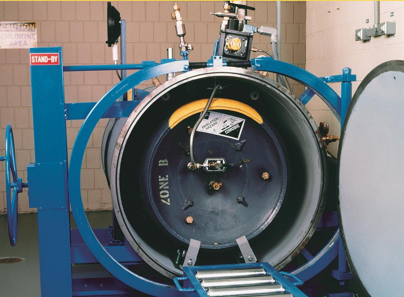
ChlorTainer is a high-pressure containment vessel into which a ton chlorine gas cylinder is processed. If the cylinder should leak, all chlorine gas is contained within the vessel and processed at a normal rate, so no hazardous waste is generated. Scrubber systems, fans, pumps, tanks, and mechanical systems are not required. ChlorTainer addresses RMP considerations, enhances site security, and provides fail-safe protection for plant operators.
