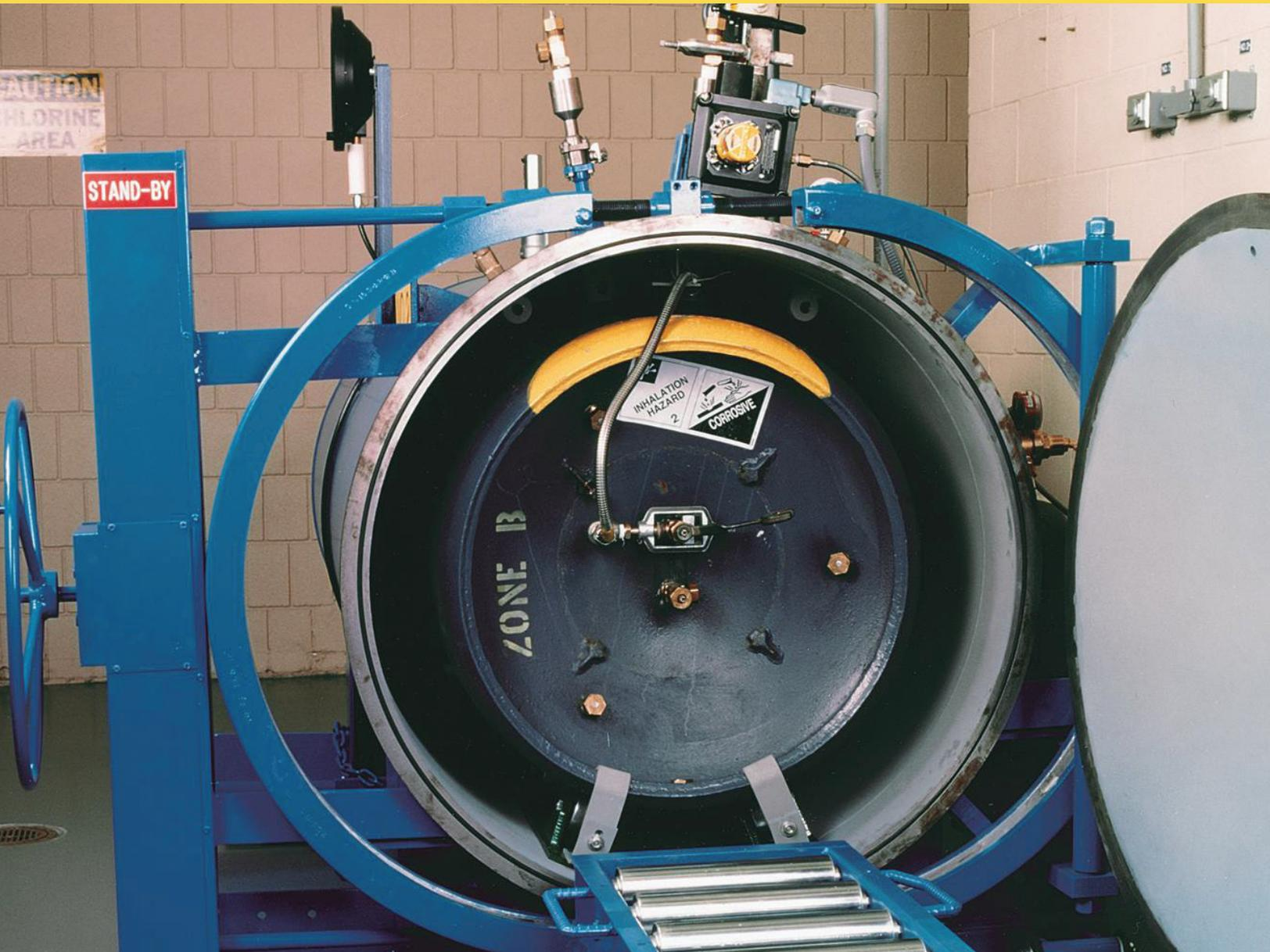
ChlorTainer is a high-pressure containment vessel into which a 1-ton chemical cylinder is processed. If the cylinder should leak, all chemicals are contained within the vessel and processed at a normal rate, so no hazardous waste is generated. Scrubber systems, fans, pumps, tanks, and mechanical systems are not required. ChlorTainer addresses RMP considerations, enhances site security, and provides fail-safe protection for plant operators.
