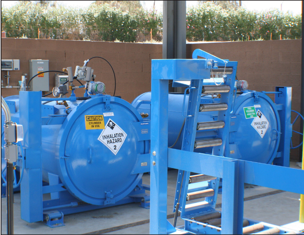
Two 1-ton ChlorTainer™ units like these, with one online and the other serving as a backup, are deployed at each of two arsenic treatment facilities (ATF's). When a cylinder switches over, a replacement is ordered for the empty. Any 1-ton cylinder with chlorine in it is always in a Chlortainer.
